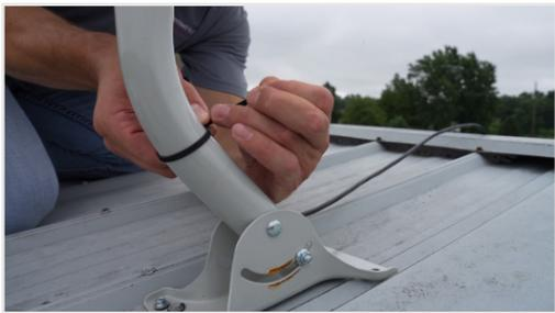
3) Using zip ties, secure the Ethernet cable to the Antenna Mast and to the structure. Do not pull too tightly, as it could damage the cable.
