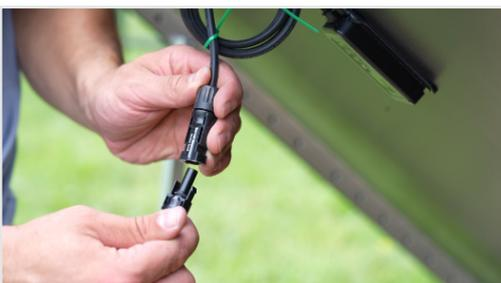
5) Using the supplied black solar panel cable, connect one end to the solar panel. You want to push the cable in until you hear a “click.” Connect the other end to each of the plugs coming out of the back of the tote.
